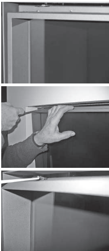
- With the hook, pull the thin, metal spring strips on the top left and right from the studs on the frame.
